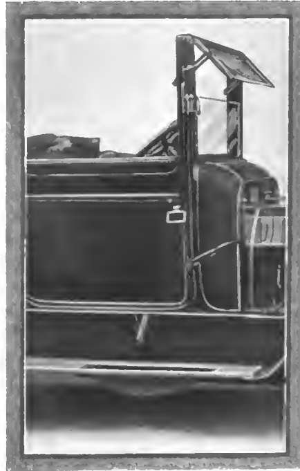
Fig. 8—Dashboard in a closed car, fitted with a glass window to permit the driver to properly see the dash fittings
